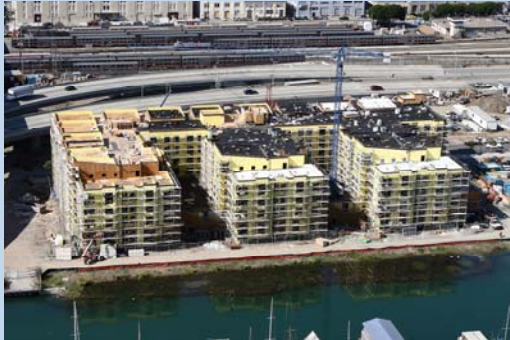
355 Berry Street, a Nibbi Bros. infill project in San Francisco
